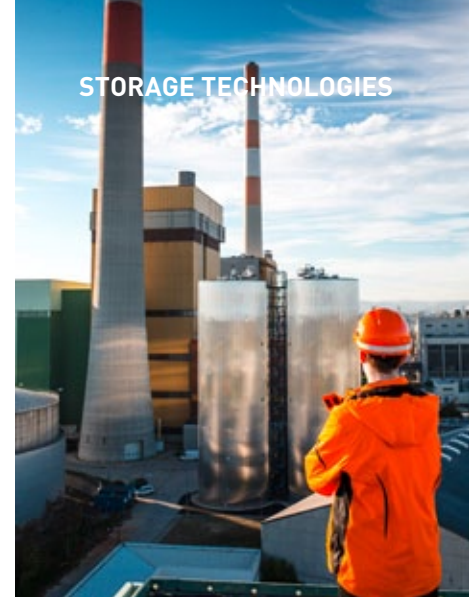
High pressure heat storage facility at Simmering power plant Photo: Wien Energie/Ian Ehm
