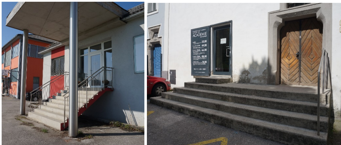
Figure 7. Elevated entrances in an area prone to flooding (left, Windischgarsten; right, Steyr); own photo 2017.
