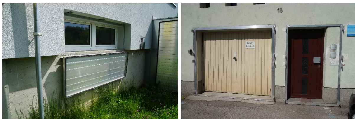
Figure 6: Possible structural protection measures: Left, a permanently installed window guard; right, mounts to hang in mobile flood protection elements which are kept nearby; own photo 2017.
