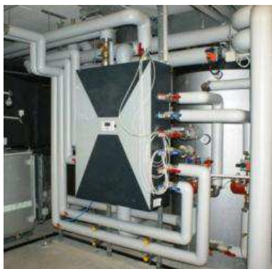
Abbildung 9: Energy Management System (EMS) (Bildquelle: AEE INTEC).
